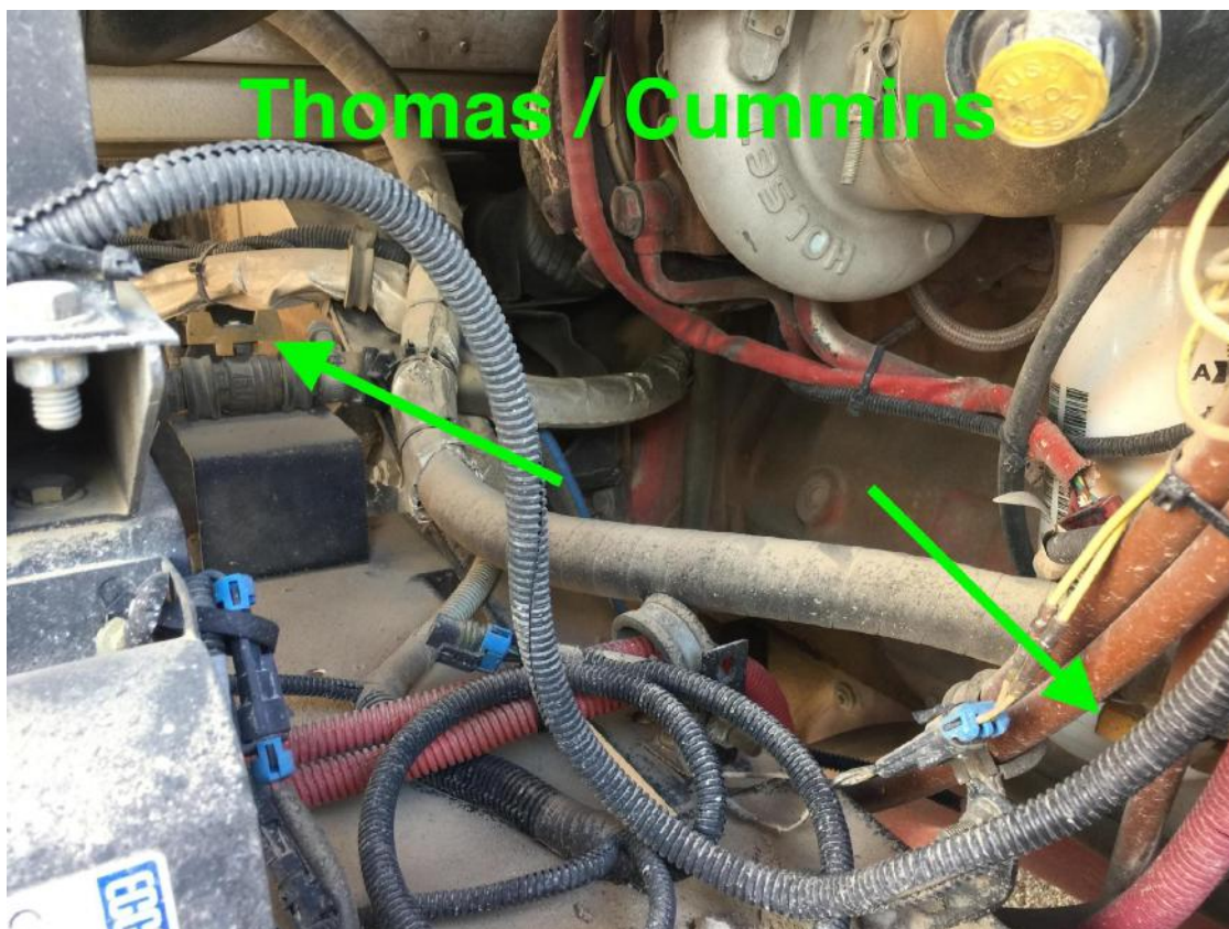
Figure 12 – Thomas Cummins Heater Valves
