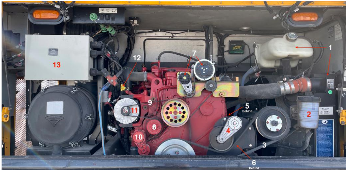
Figure 7 – Engine Compartment Inspection
