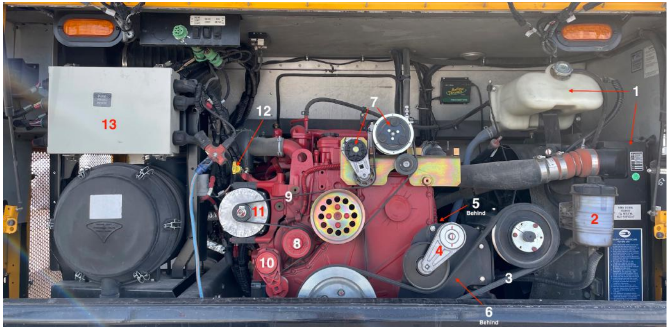
Figure 7 – Engine Compartment Inspection
